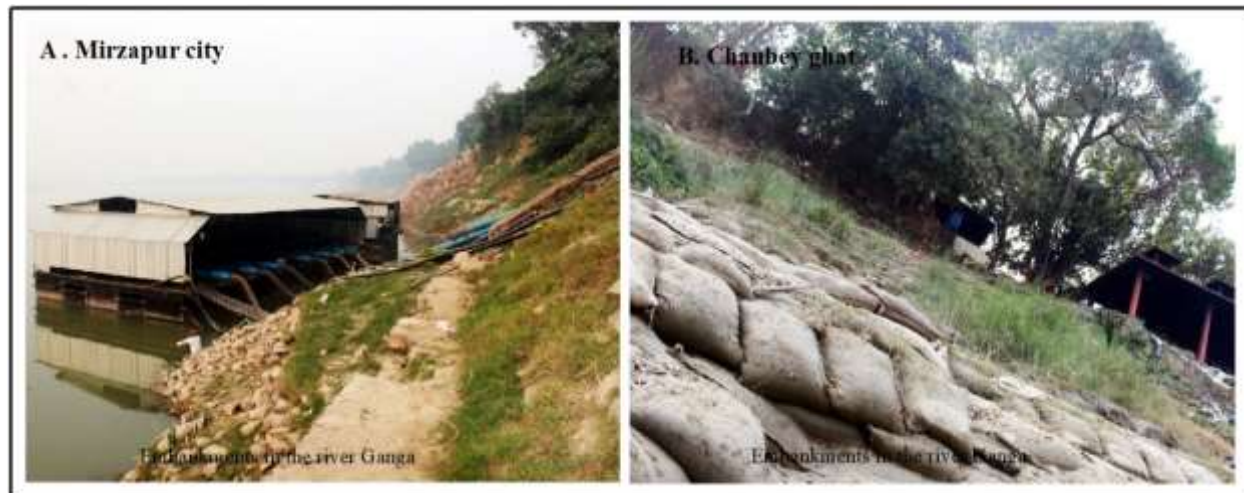
Plate: 10 Photographs of the embankment of the study area. (A) view of the sandstone embankment at Mirzapur city. (B) view of embankment made by sand and stone at Chaubey Ghat.
